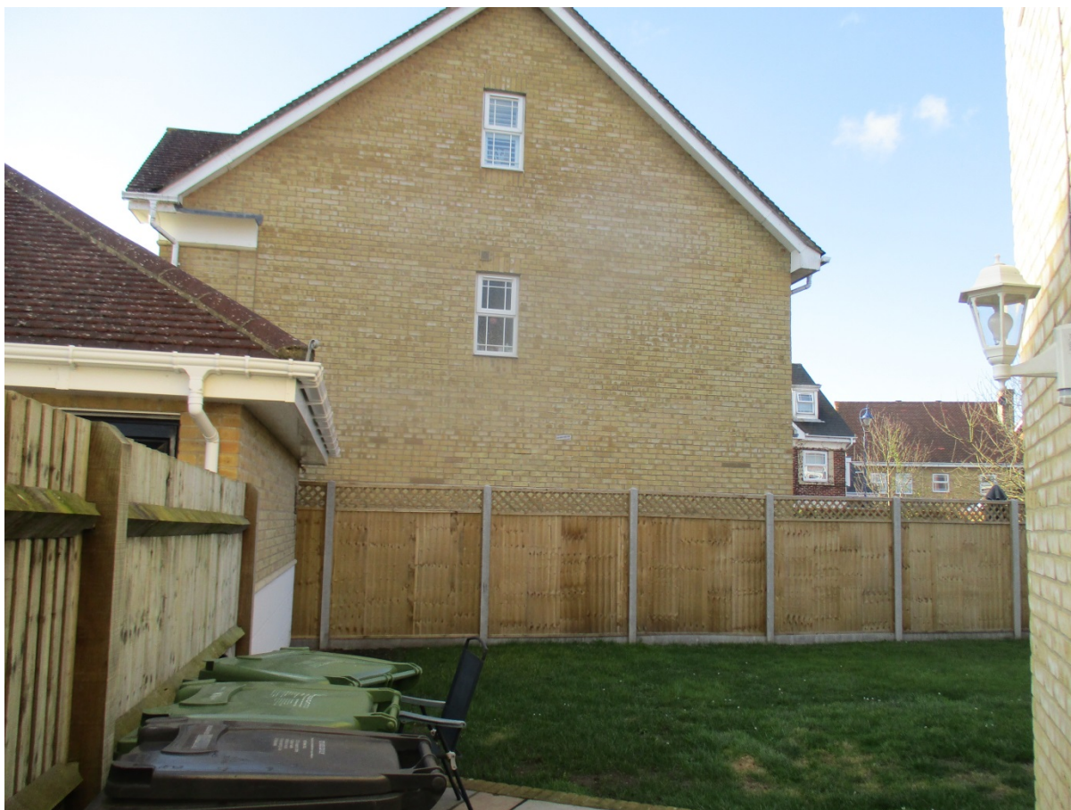
View from No.9's rear garden looking towards the flank wall of No.16.
