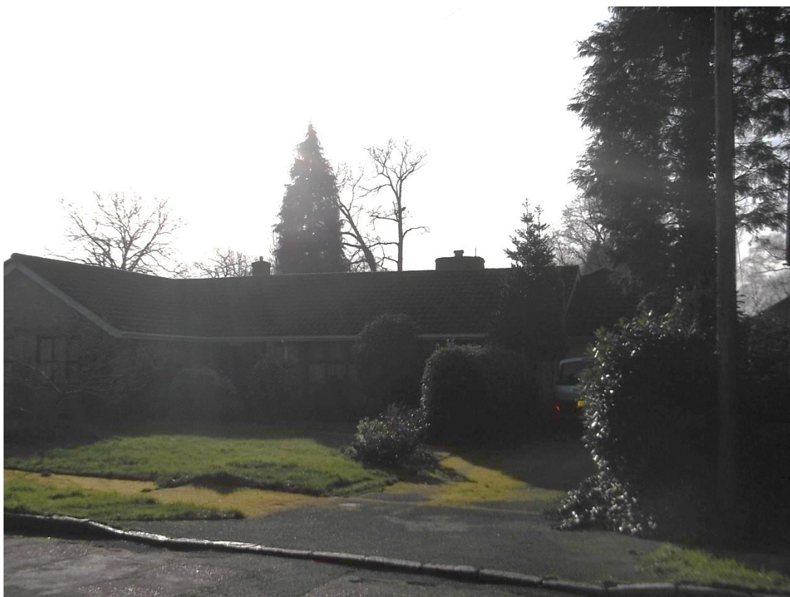
View from street of Tidybrook
